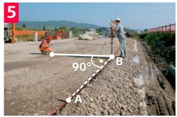
Guide the reflector carrier into and along the line of sight of the telescope.
