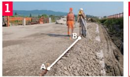
Setup and level the instrument over point B.
