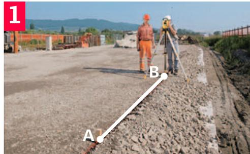
Setup and level the instrument over point B.
