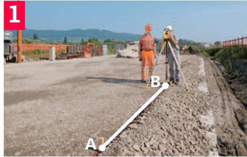
Setup and level the instrument over point B.
